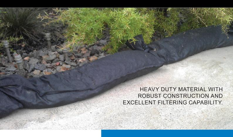
Silt socks are a cost effective, temporary solution to control water movement, minimise site wetness and reduce soil erosion.
